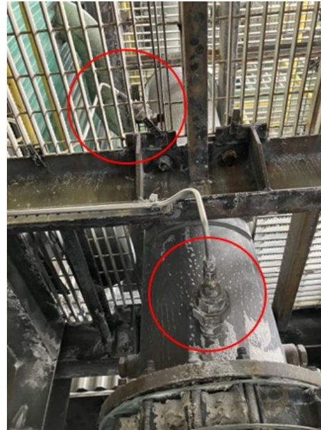
Figure 10. Nozzles location in the column.
