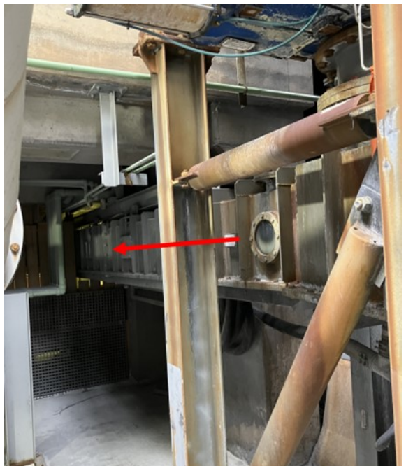
Figure 3. Siphon under center passage.
